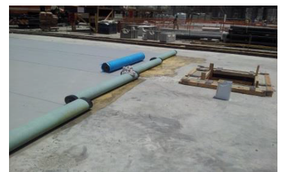
Adjacent rolls of Proofex OFB with hot-air welded overlaps
