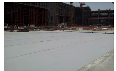
Proofex OFB membrane fully bonded to the concrete substrate
